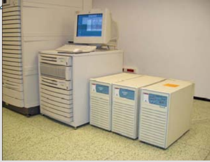
Central processing unit of SAFIR 3000 system
