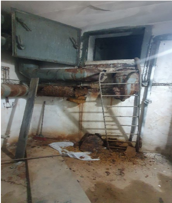
Ministry of Transport - deficiencies in the filter- ventilation installation, emergency exit
